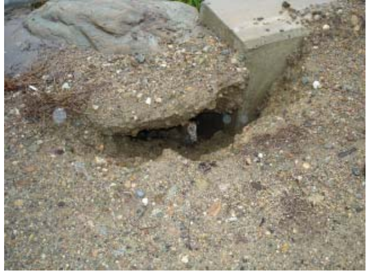
Photo 5 — Short-circuiting of drainage structure
