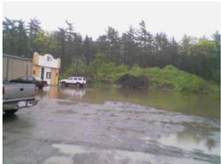
Photo 8 — Buried catch basin resulting in severe flooding
