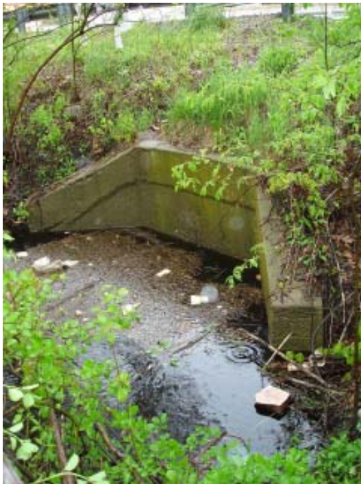
Photo 6 — Submerged outfalls
